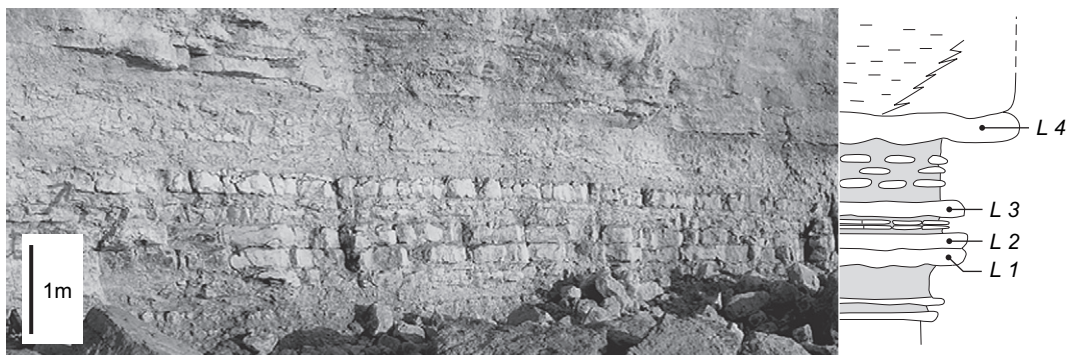
Fig. 2. View of the Belette outcrop at South of the Pointe-du-Chay and schematic stratigraphic column. Layers 1 to 4 are composed of fine grain carbonate rocks (mudstones) included in more argillaceous layers. Stratabound joints are limited to the carbonate beds only.
